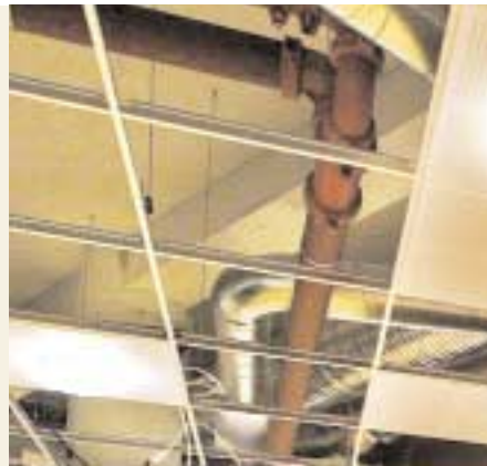
Sonebasert el-kraft installert over himlingen.
